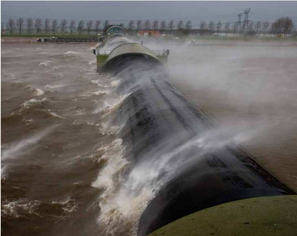
Figure 11-2: Ramspol Storm surge barrier in operation (credits: Ministry of Infrastructure and Water Management, The Netherlands).
